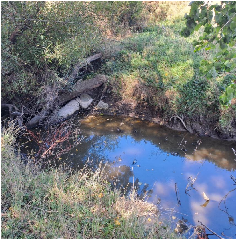
Figure 6. Photo of a section of John Creek with signs of active erosion, dated February 2024
